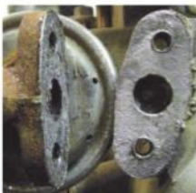
1 Expose clogged EGR port
