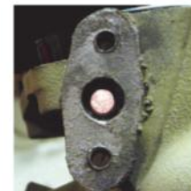
3 Use steel brush or pick to clean remaining deposits
